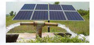
The research activities on this area concentrates on application of Standalone Solar Photovoltaic Systems in various rural development activities like water pumping, solar refrigeration, Water purification etc.
